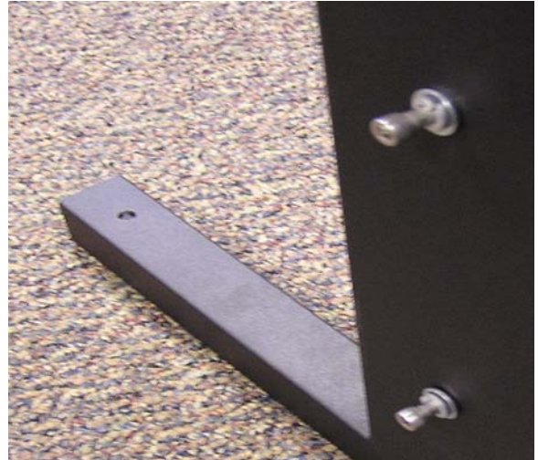
Figure 2: Bolt with washer and lock washer
